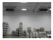
refrigerated spaces. In particular, the FZBT-TL-400WA3 can be mounted at any angle to provide illumination in high ceiling facilities. A single 400-Watt Freezer-Bright<sup>TM</sup> generates more visible light than four 400-Watt metal halide high-bays for more than 80% in electricity savings including ballast overheads. The
